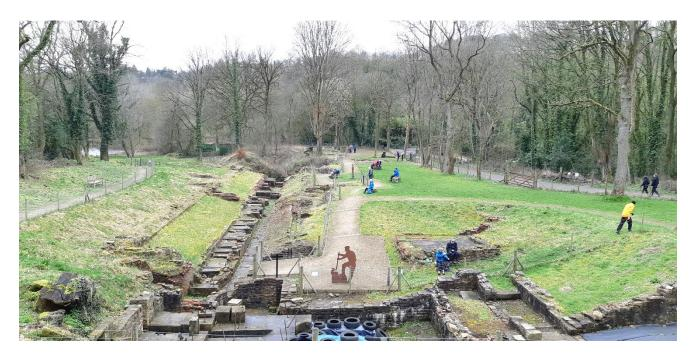
Mellor Mill was built in 1790 and was, at the time, the largest cotton spinning mill in the world! At its peak in 1804, 550 people were employed. For 60 years the mill was water driven, the first prime mover was the "Wellington Wheel", 22 ft. in diameter X 17 ft. wide. The wheel pit has been exposed and viewing platforms provide easy access. In 1815 the "Waterloo Wheel" was added to provide more power. The whole Mellor Mill and
